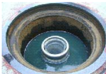
This spill bucket contains liquid.
